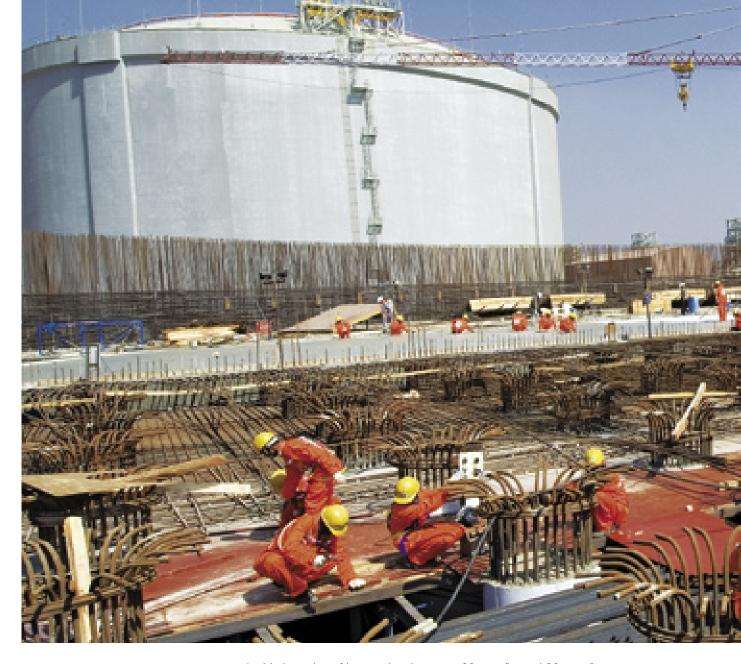
double integrity refrigerated tanks have a height of 63.5 m at the topmost point of the dome. The internal diameter of the tank is 79 m making it almost as big as a full sized football field. The working height of the tank is 37 m. Each tank rests on as many as 578 bored cast insitu piles, each having a diameter of 1 m, with a depth 36 m.
